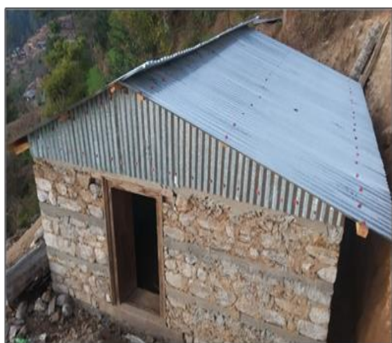
Newly constructed earthquake resilient house of Bir Bahadur Thapa
